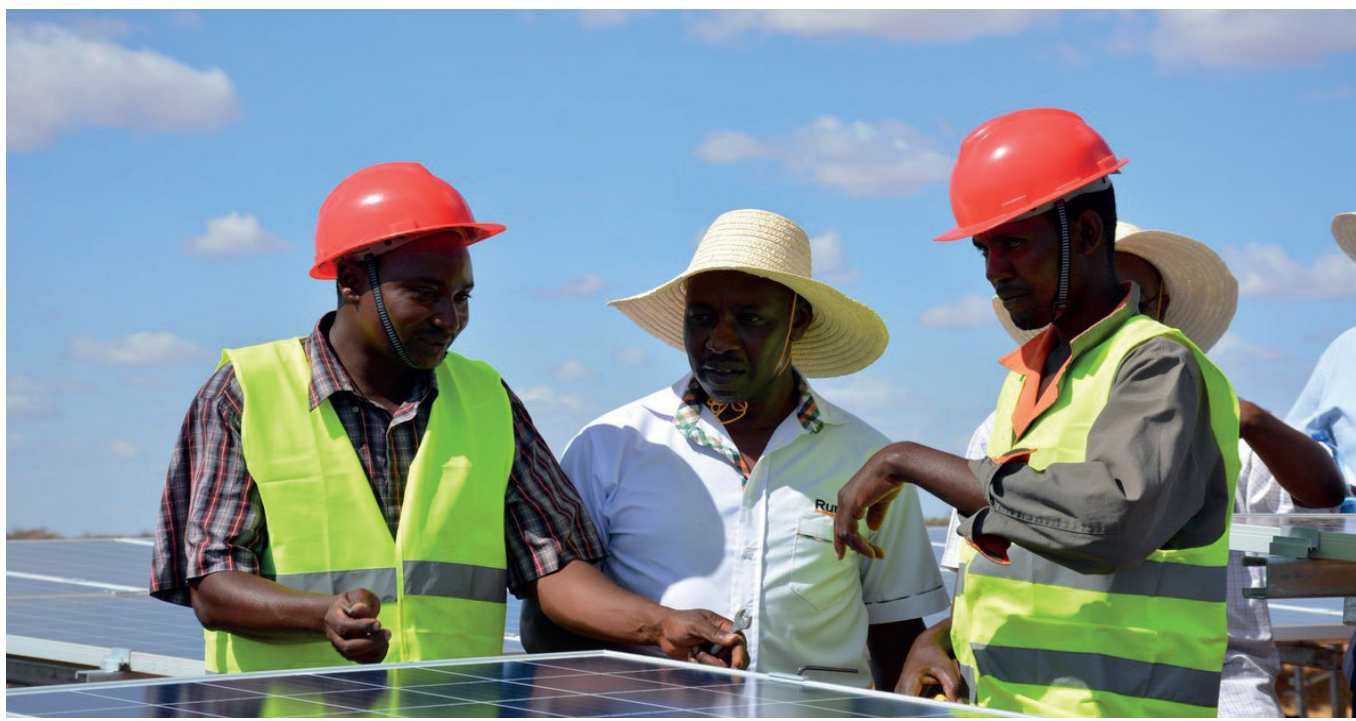
REREC CEO Peter Mbugua (Center) with the Corporation's contractors in Garissa County. The Operations and maintenance of the Ksh 13.5 billion Garissa Solar Power plan constructed by REREC will now be managed by KenGen
