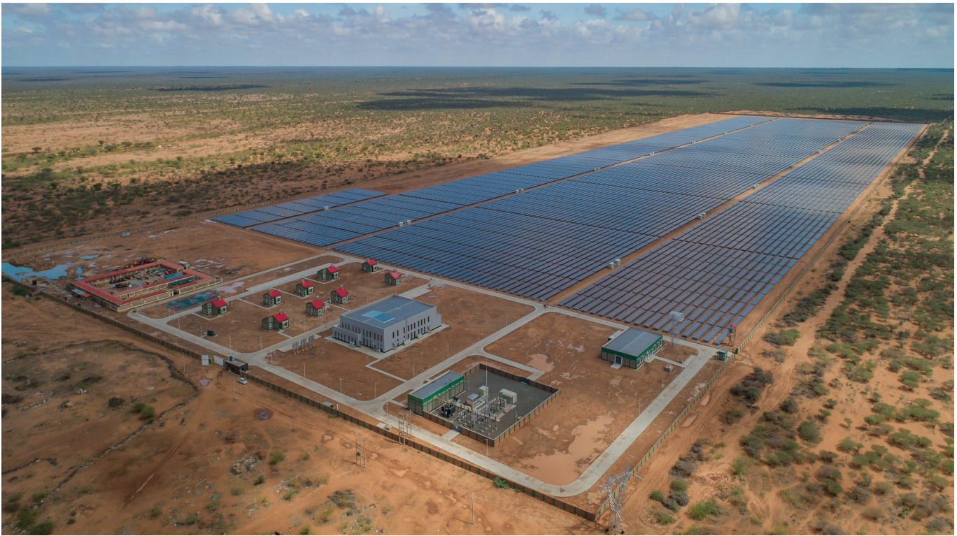
Garissa Solar Power Plant built by Rural Electrification and Renewable Energy Corporation (REREC).
